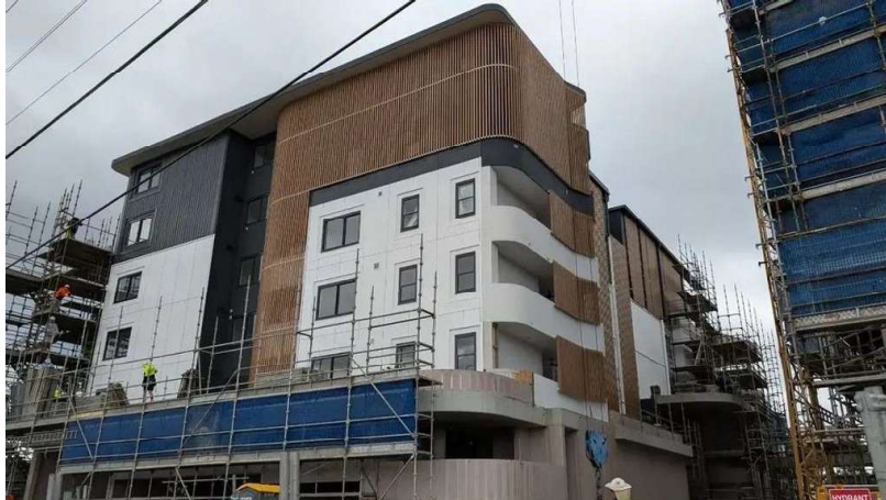
Kokomo under construction in a photo from September 2024.
